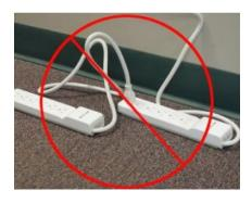
Extension cords or long equipment cords can be mounted overhead or secured on the floor with a non-conducting bridge. They must not run along walkways, through walls, or above ceilings. Protect power strips from water or chemical spills and splashes by mounting them above ground level.
