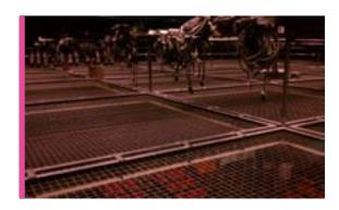
The tension grid is modular wire grid system that provides access to theatrical lighting, audio cables, loudspeakers, and stage rigging. Any edge of the grid that is not attached directly to a wall must be equipped with guardrails.
