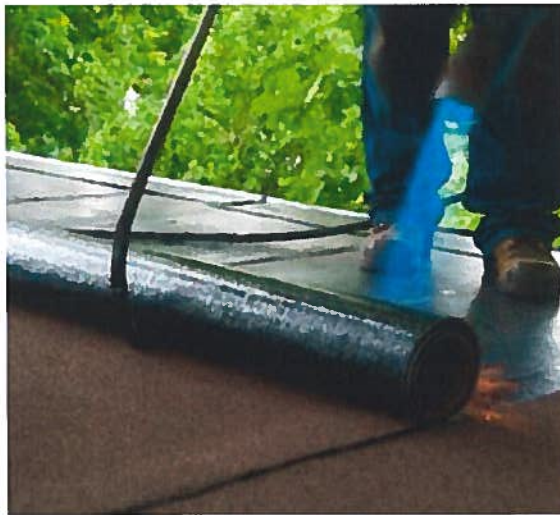
Torch-Applied Roofing Operations
