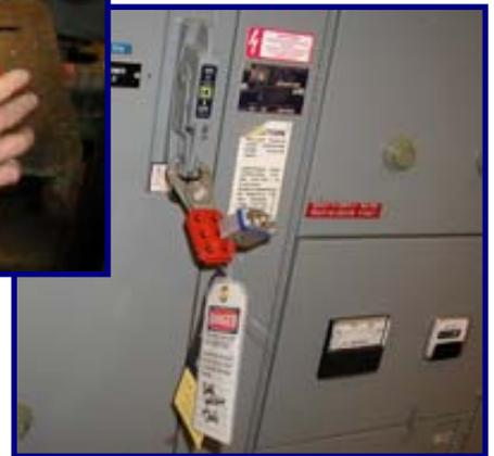
Above right: Locks are necessary to prevent unauthorized changes to machine power status. Tags are useful for identifying why something has been de-activated, how long it will be out of service, and who to contact regarding the progress of repairs. Only the worker who applied the lock is allowed to remove it!
