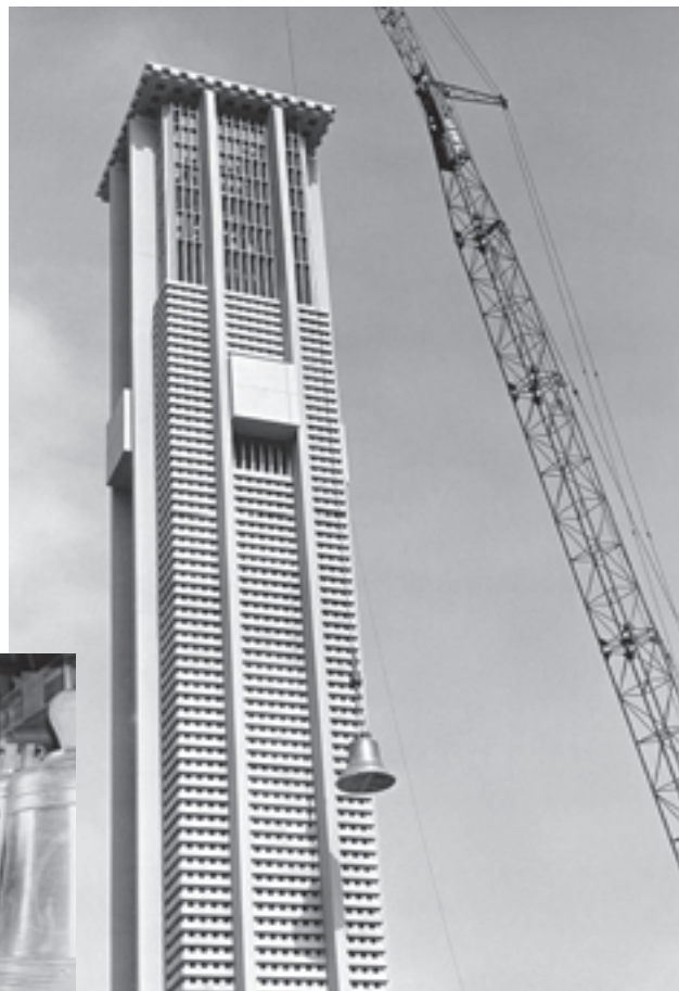
Construction of the Carillon Tower
