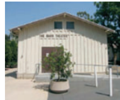
Barn Theater – West Façade
