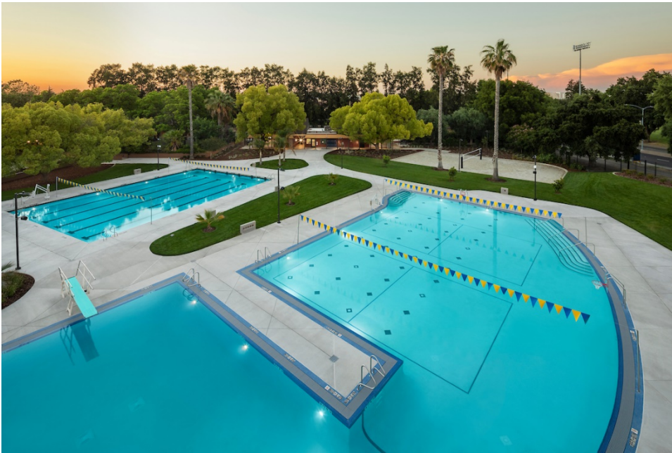
Photo: UC Davis Recreation Pool Renovation
