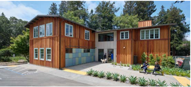
UC Berkeley, Dwinelle Annex
