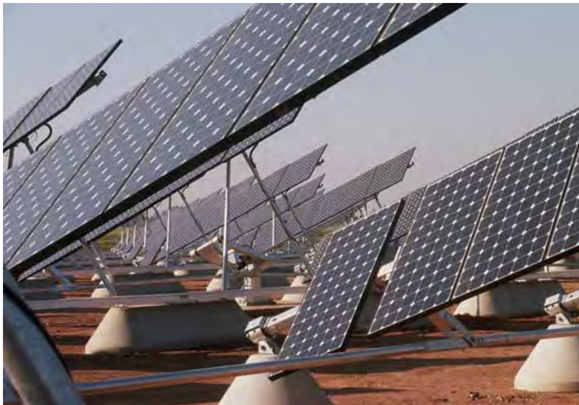
UC Merced's 1 MW solar array.
