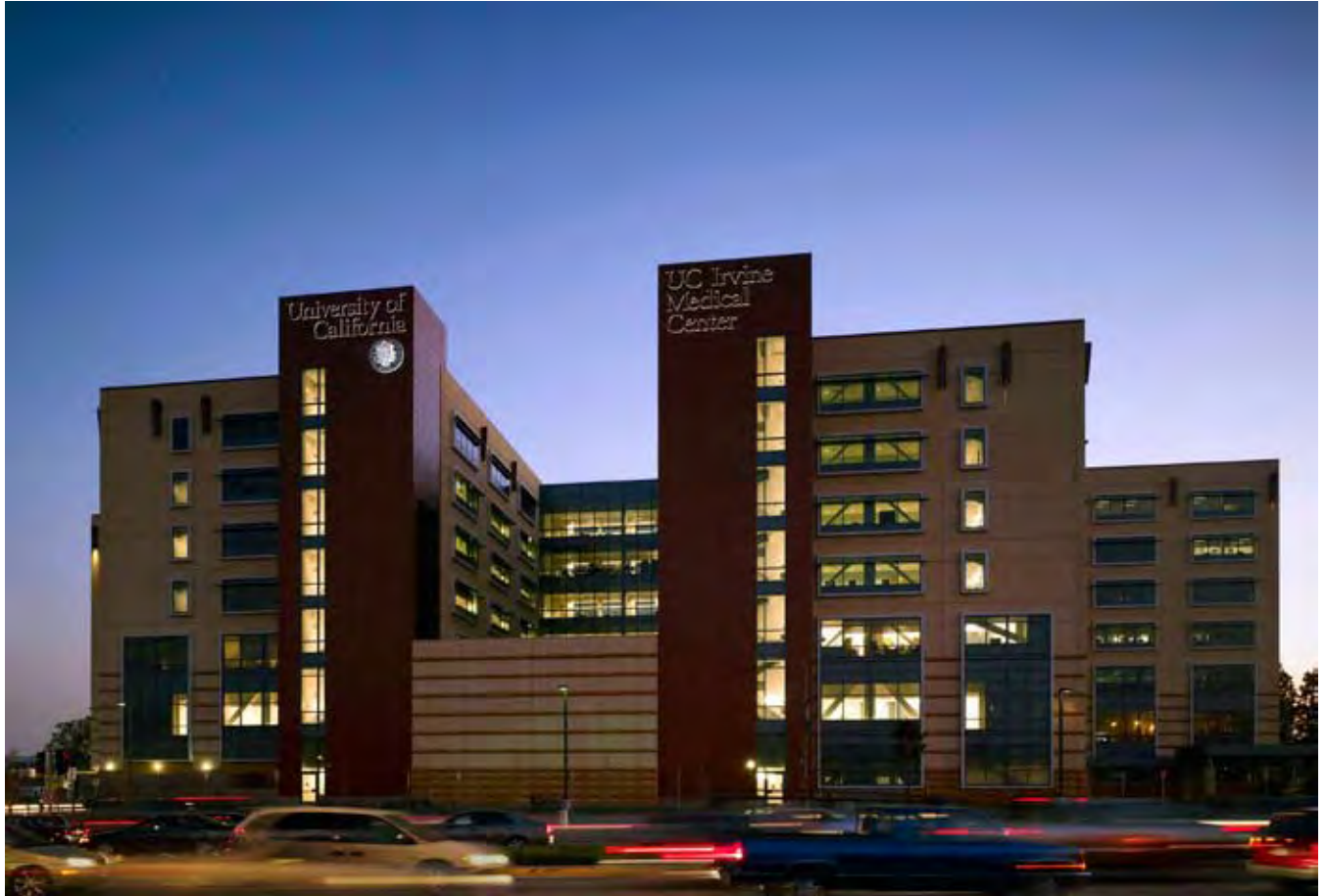
The UC Irvine Douglas Hospital (Photo by Nick Merrick, Hedrich Blessing Photographers)
