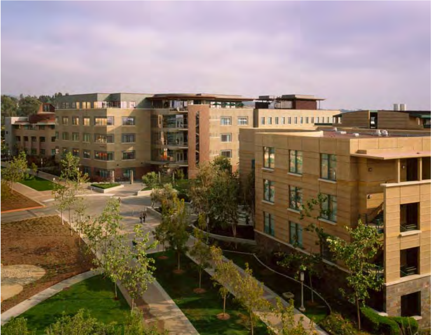
Croul Hall, Natural Sciences II, and Natural Sciences I (left to right). (Photo by Nick Merrick, Hedrich Blessing Photographers)
